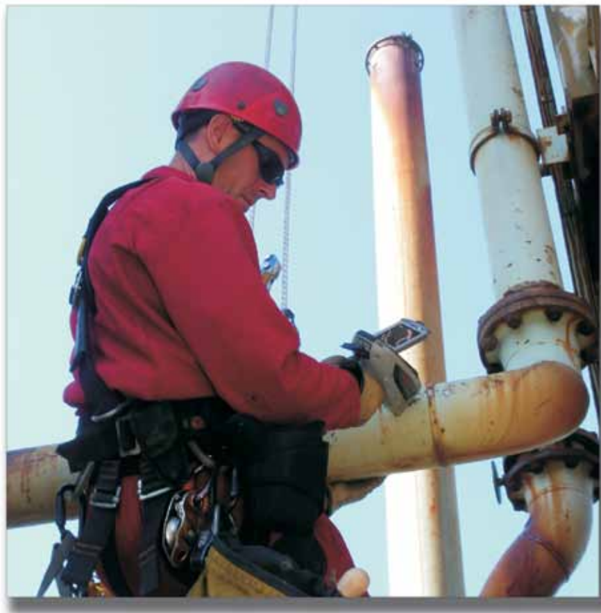
An inspector uses a handheld XRF analyzer to check weld chemistry on an existing piping system as part of a retroactive PMI program in accordance with API RP 578. Photo courtesy of Thermo Fisher Scientific.
