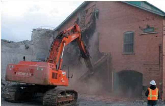
Demolition of the power house.
