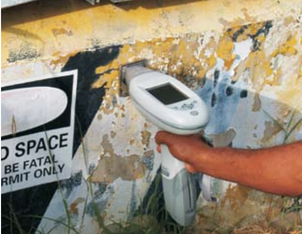
Industrial lead paint measurement for site assessment and worker protection.
